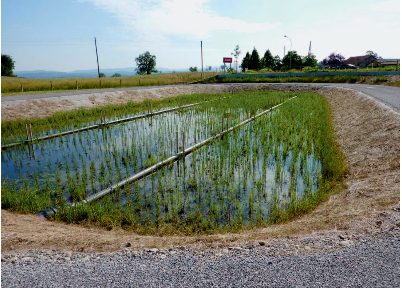
2 | SABA Chringelbach, Forchstrasse (Foto: ilu AG). 2 | SETEC de Chringelbach, Forchstrasse (photo: ilu AG).
